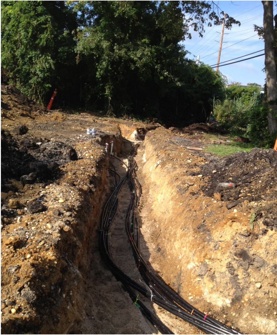
Trenching and installation of oxygen supply piping at 87 Community Road
