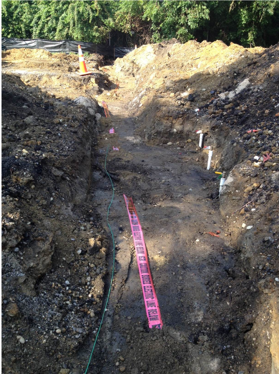
Toner wire and demarcation tape installation at 87 Community Road
